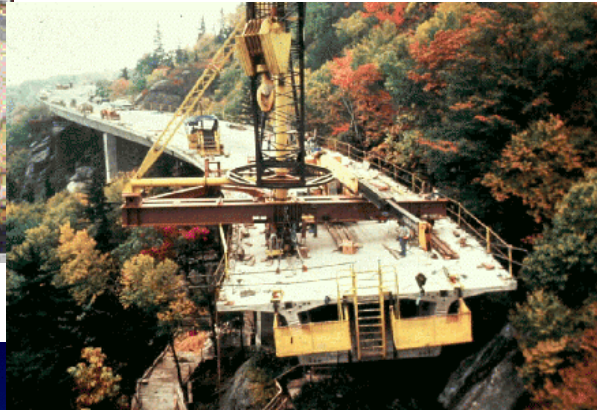
Note the use of trapezoidal box girders
