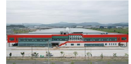
산업설비 (Industrial Facility)
